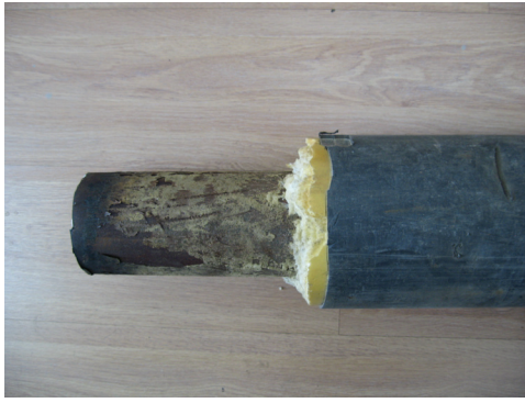
Fig. 1. Corrosion pre-insulated pipe.
