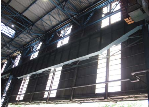
Fig. 1. Crane girder structure with trapezoidal variable cross-section.
