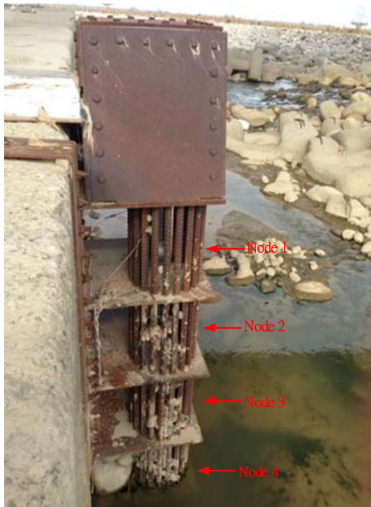
Fig. 12. The results of bridge scour in the field.
