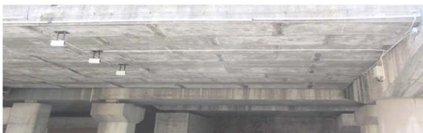
Fig. 9. A photo of the bridge after all the sensors were installed.
