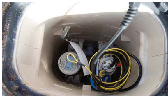
Fig. 5. Acoustic sensor for Primayer geographically distributed monitoring system.
