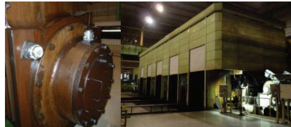
Fig. 8. Cold strip mill application environment.
