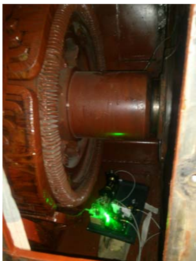
Fig. 7. Experimental setup for detecting the change in coil current in the field winding of a DC motor.
