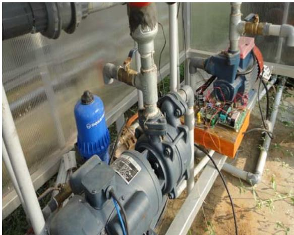
Fig. 9. Relays controlling motor.
