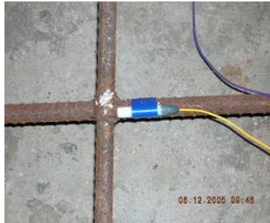
Fig. 2. Installation of OCP sensor over the rebar.
