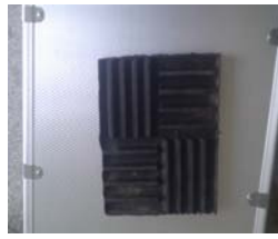
SD shear vibration isolator
